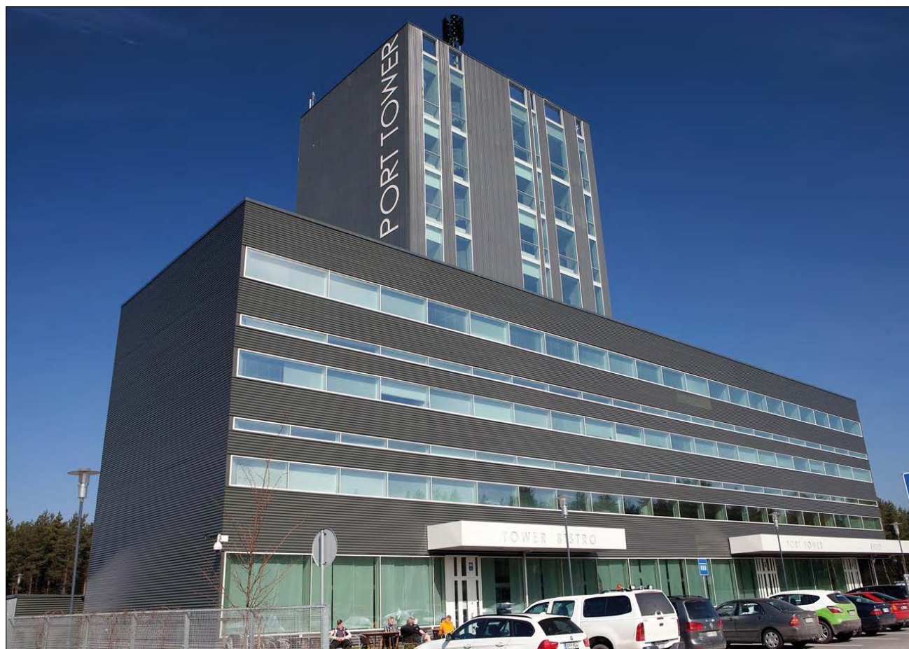
The Port Tower has been built on the new port road. Офис-центр Port Tower построен у новой портовой дороги.
